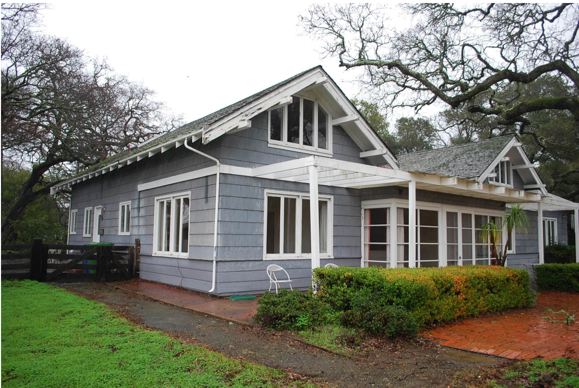
View looking SE at north and west facades
