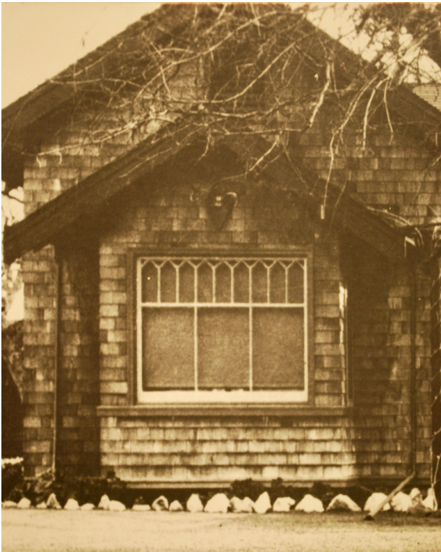
This photo is most likely of the west side, but this is not certain. Note lack of purlins in main gables.
