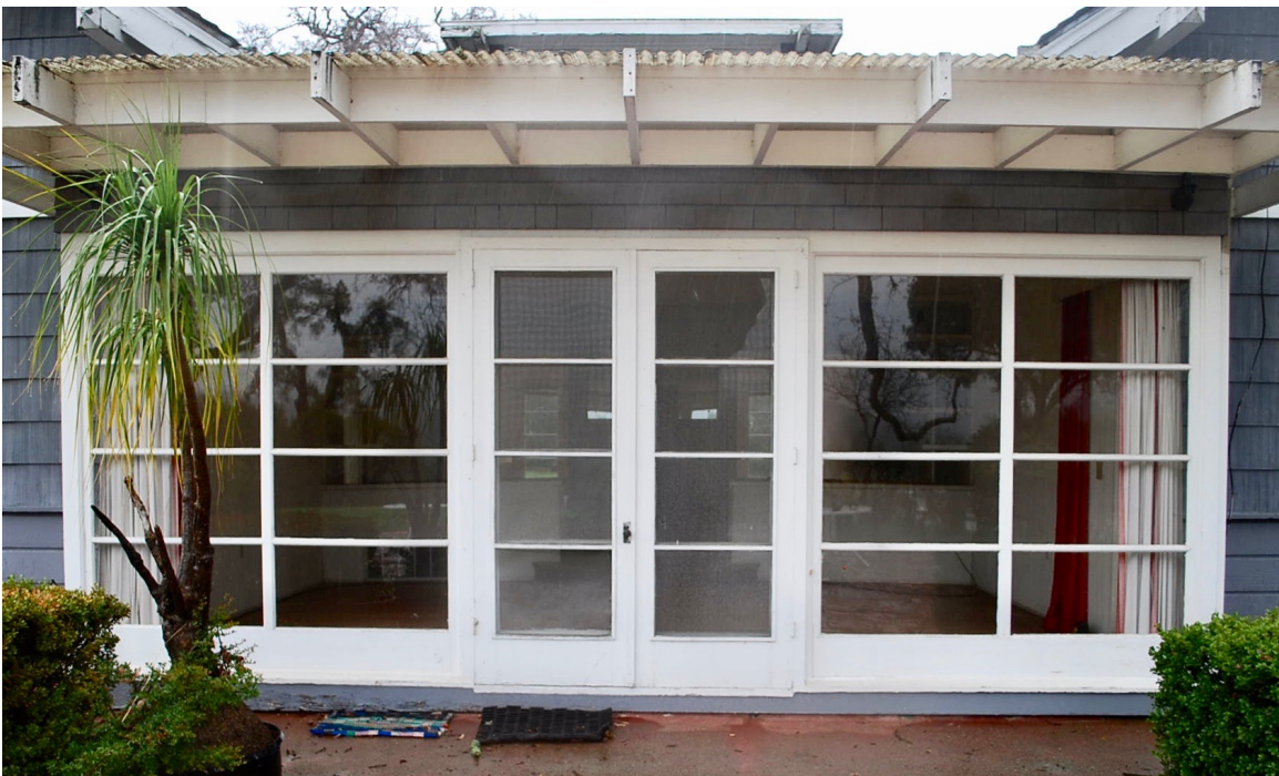
Entrance pavilion, west facade. Paired windows flank central doors.
