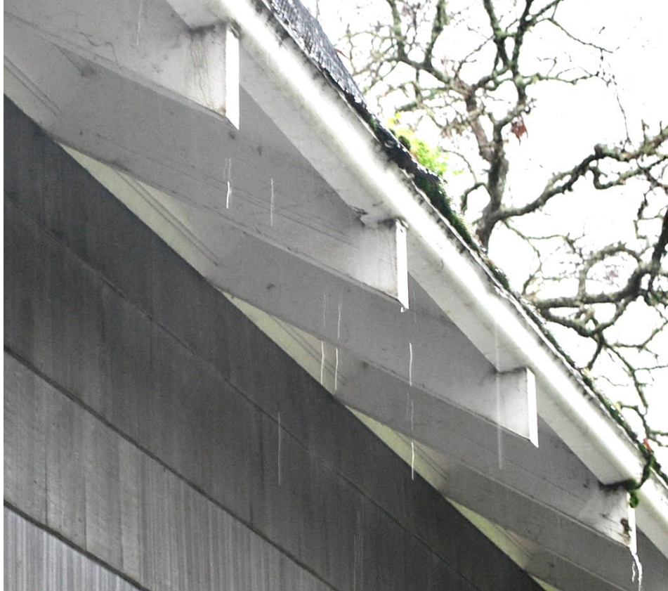
At left: Eave with exposed rafters, north facade.
