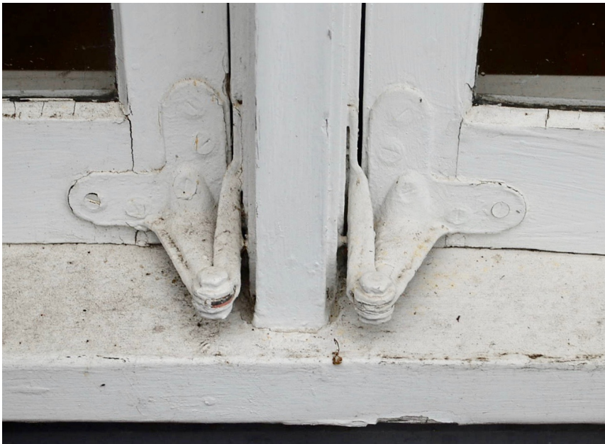
Paired casement windows, with detail of hardware.
