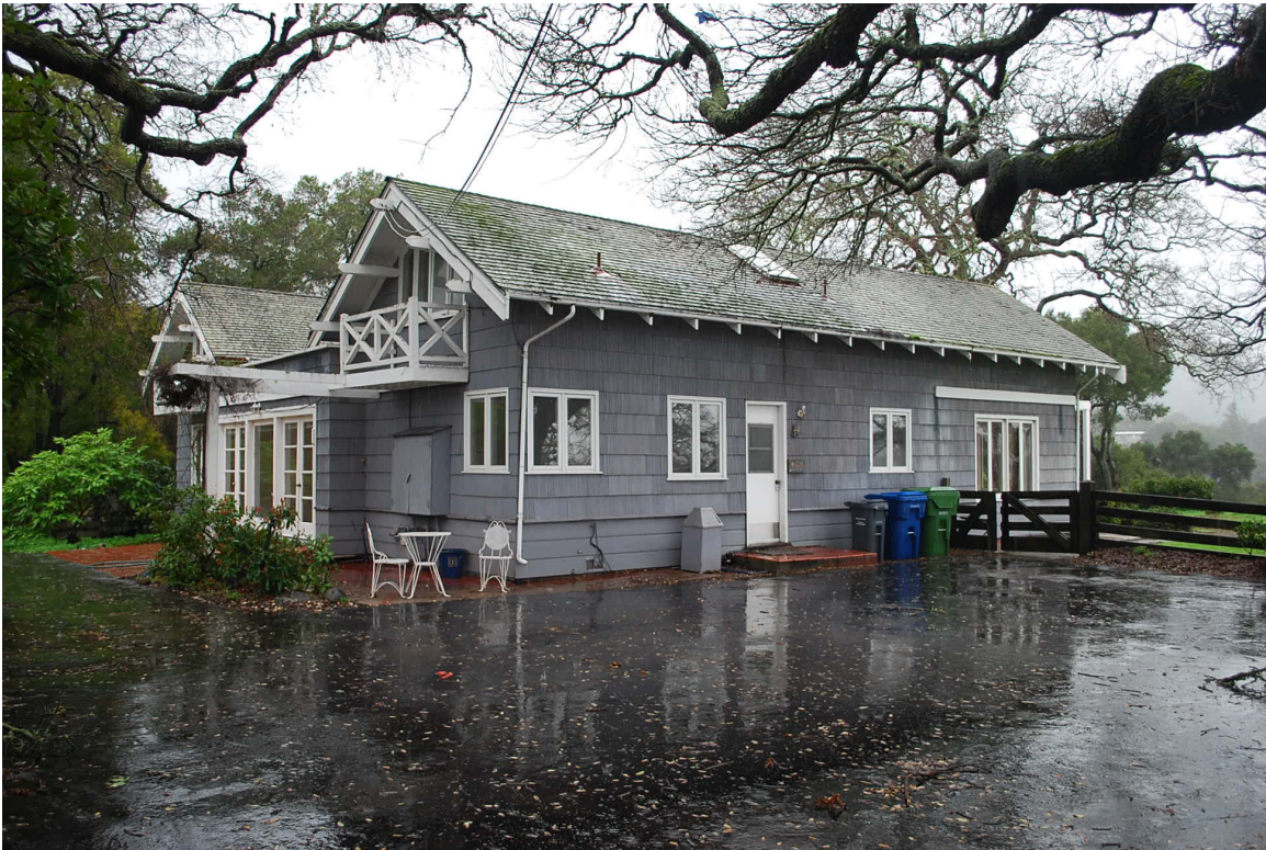
View looking SW at east and north facades
