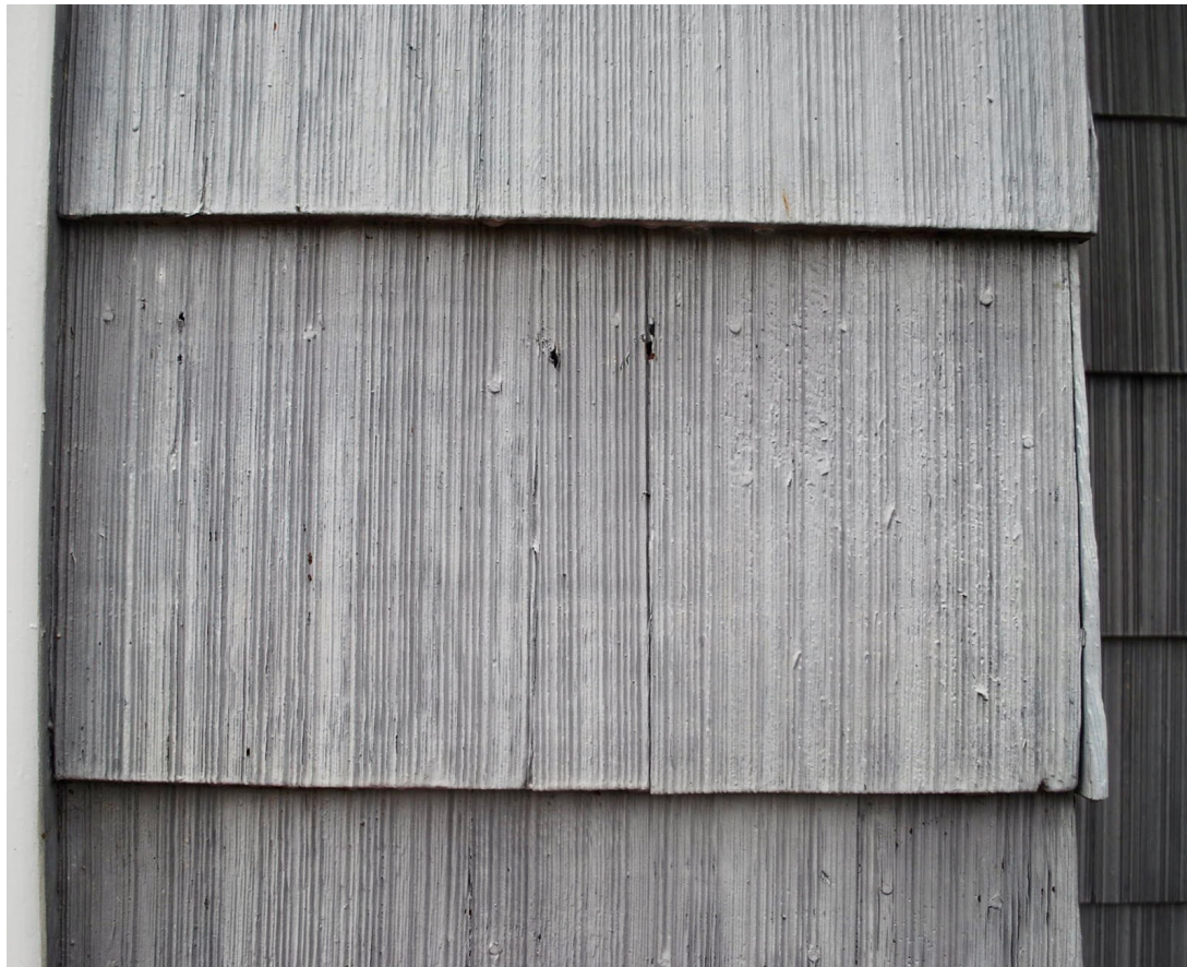
Wooden shingles. Note grooves that were added for texture in the milling process. These shingles are wider than typical cedar shingles of the 1890s-1910s. These are similar to shingles used in some suburban houses during the late 1940s and the 1950s.
