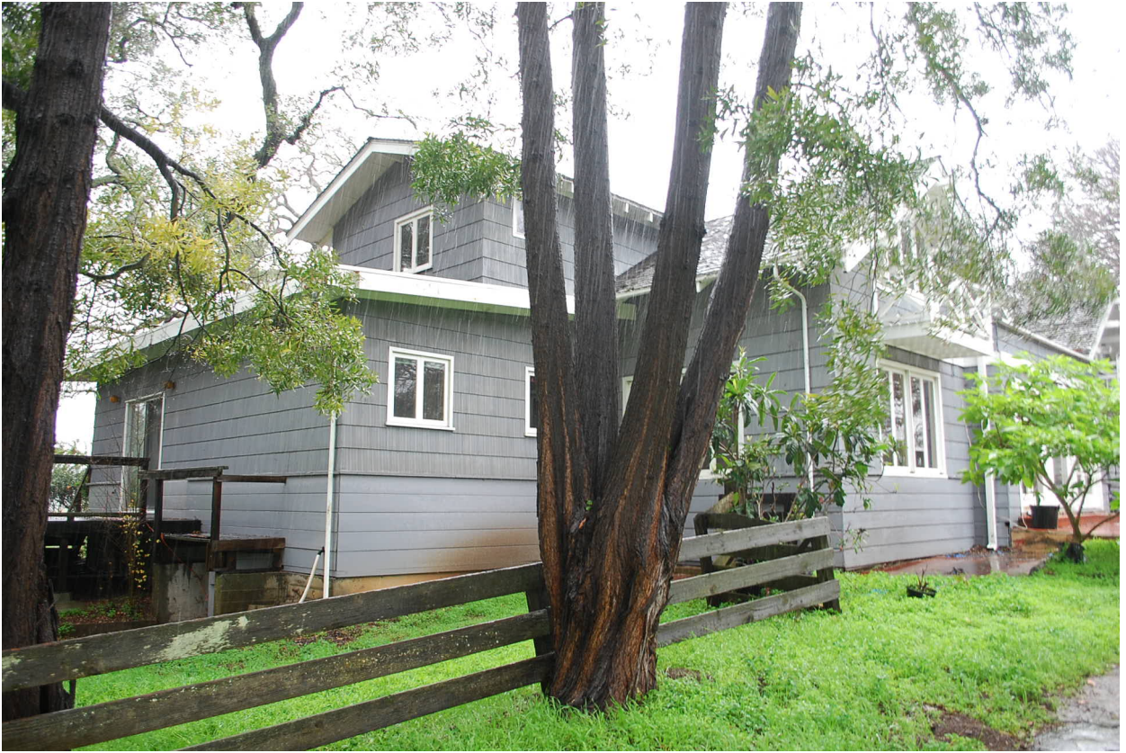
View looking NW at the south and east facades
